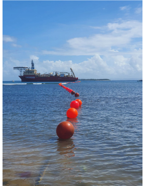
23/12/20 – CS Fu Hai landing SCiP cable at Matnog (@philBE2 on twitter)
