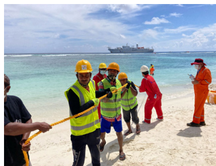
Landing Operation of MSC cable in Hulhumale'
