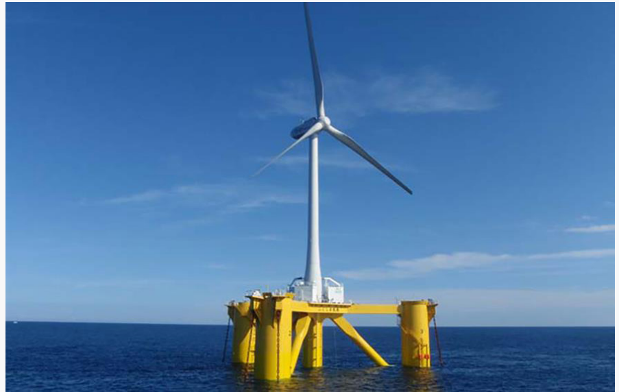
The 2MW Hitachi test turbine on a floating platform off Fukushima
