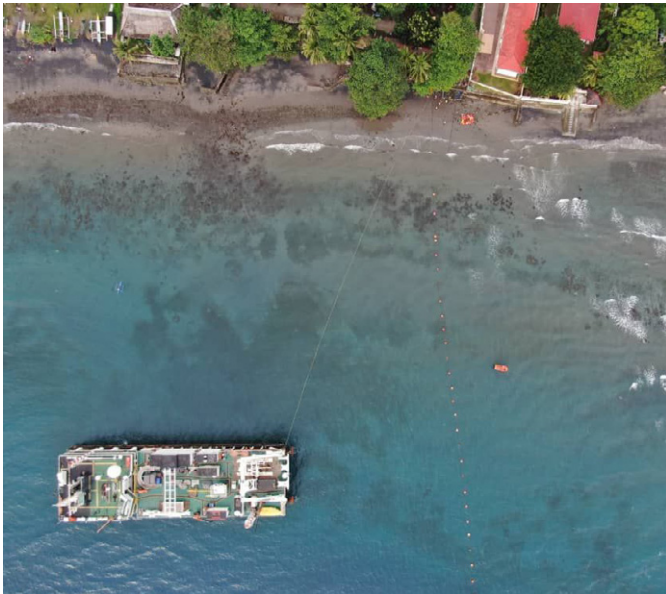
01/01/2021 – Direct shore-end landing for SCiP Segment 1.7 at Dumaguete
